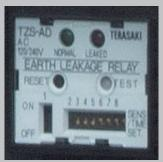
The earth leakage relay detects insulation failure, and automatically cuts the circuit off to prevent electrical shock.
